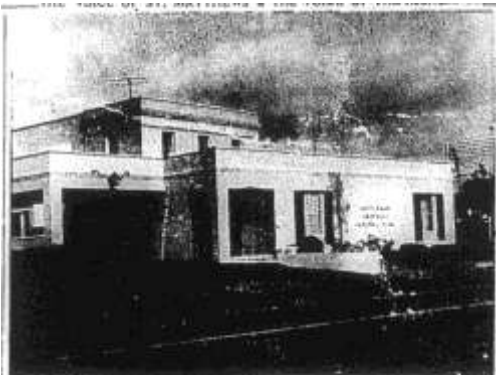
The appearance of Ratterman Brothers Funeral Home, 3711 Lexington Road, after renovations and an addition to the front. Added were two new parlors, a casket display room, lounge and addition to a chapel.
